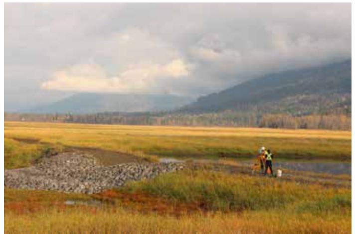
Cartier Bay project location after work was completed.
